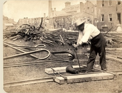
Railroad construction worker straightening track, by Andrew J. Russell, United States Army, Railway Service. 1862/3 Library of Congress
