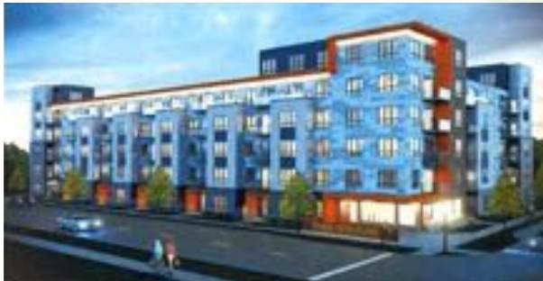
ALASKA Minnesota: West Side Flats
