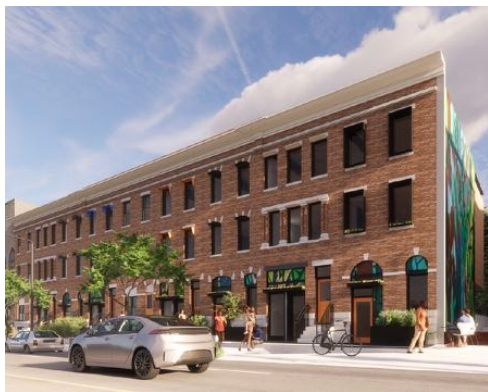
1600 North St Baltimore, MD 17 units, Passive House, NZE
