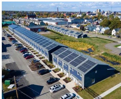
Parade St. Commons Erie, PA 40 units, Passive House, NZE
