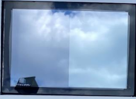
GL-1: VE-1 59 100 WITH 1/4" HEAT STRENGTHENED FLOAT GLASS OUTBOARD LITE, 1/2" AIR SPACE, 1/4" FULLY TEMPERED INBOARD LITE ON CLEAR.
