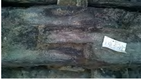
Above left: An intact mortise and tenon joint from above.
