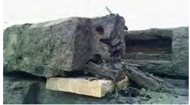
Above right: Detail of a mortise and tenon joint discovered while unloading the warehouse at the MAC Lab. Note the peg holes that run through this piece that would have secured the joint. Because of the dirt covering these beams, we had not previously seen this architectural feature. As the wood is cleaned at the MAC Lab, we expect to learn more about the architecture of this building.
