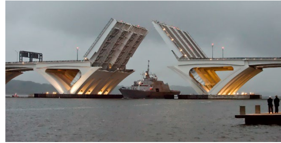
Woodrow Wilson Bridge - Foundations Oxon Hill, MD
