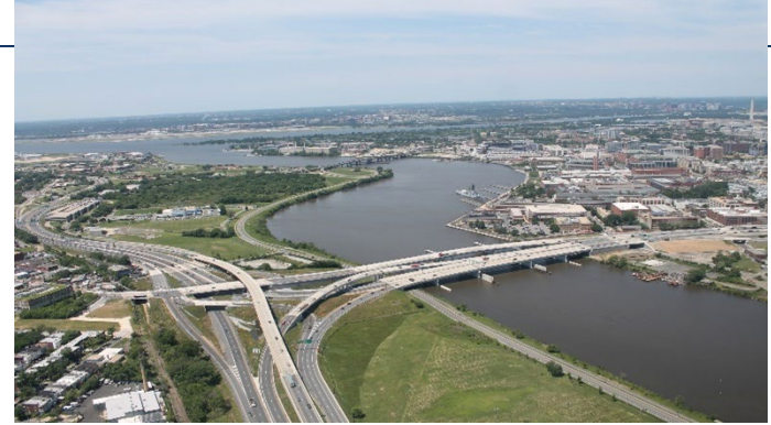
11th Street Bridges Anacostia, Washington, DC
