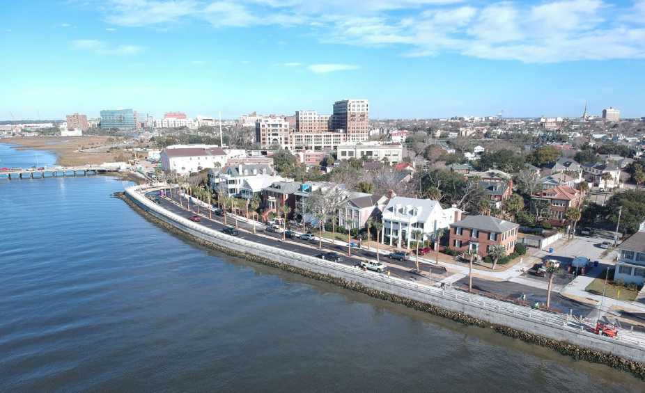
Low Battery Seawall Project Charleston, SC
