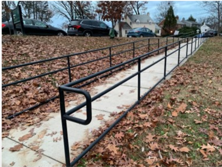
Beverly Park ADA Accessible Concrete Ramp with Rail
