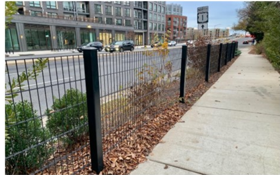
City of Alexandria standard metal fencing, Powhatan Park
