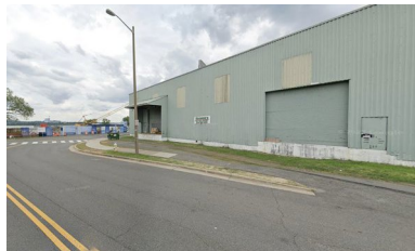
Robinson Terminal North warehouse at North Union and Pendleton streets in Old Town.
